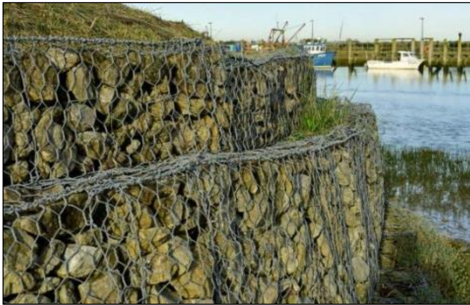
FIGURE 3: EXAMPLE OF A GABION RETAINING WALL
