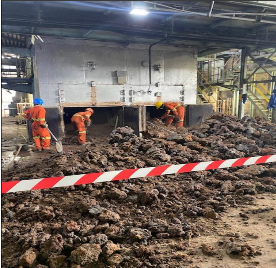
FIGURE 5-1: IMAGE OF BOTTOM ASH BEING EXTRACTED FROM THE COMBUSTION CHAMBER
